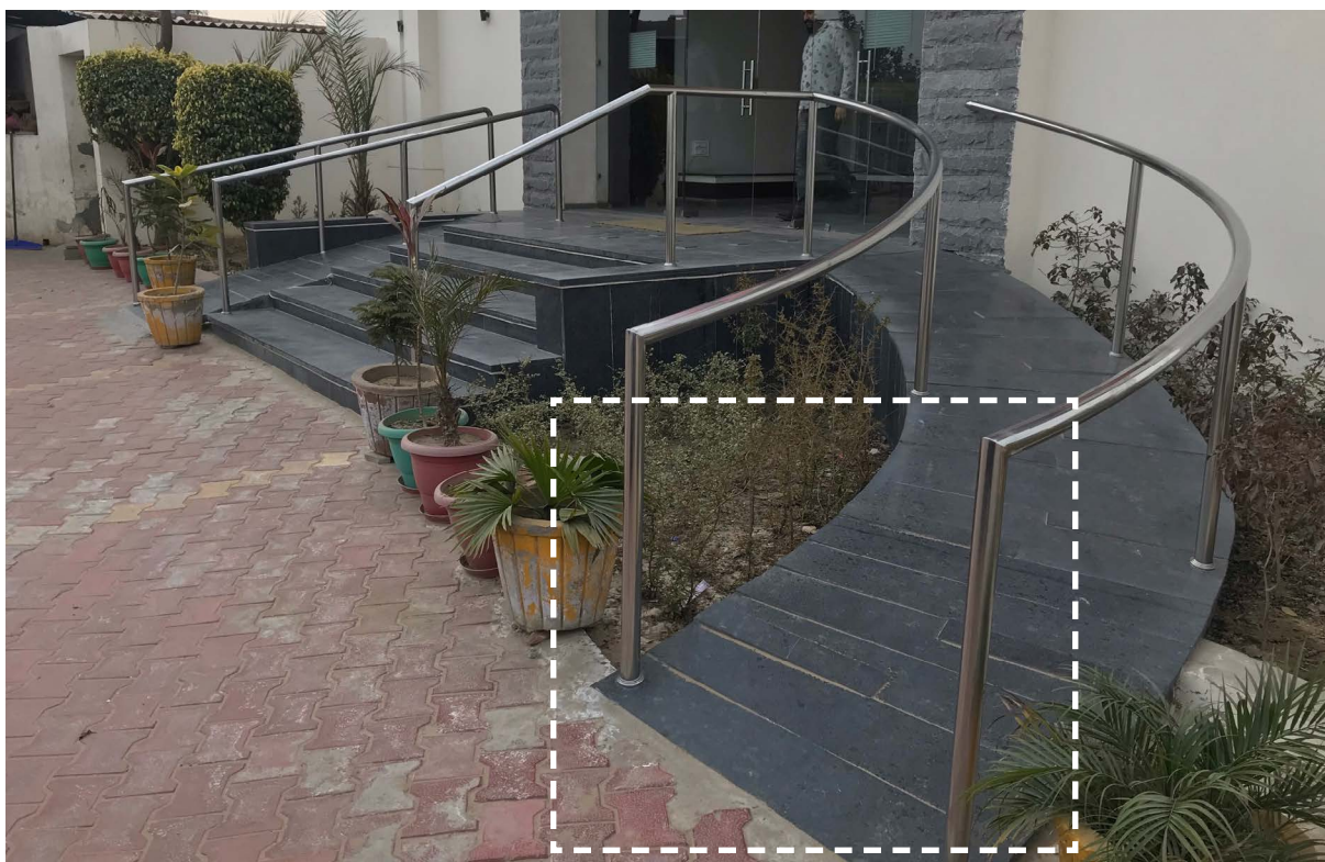
Image 2.9 Curved ramp with improper detailing and design
