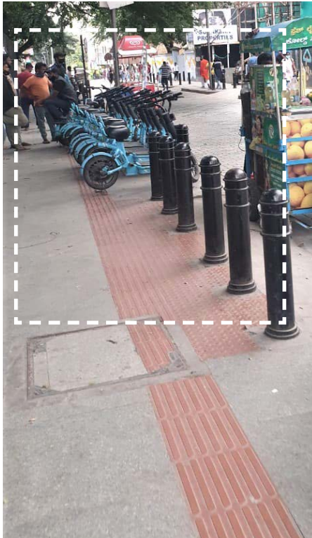
Image 2.21 Obstructions on tactile pathway
