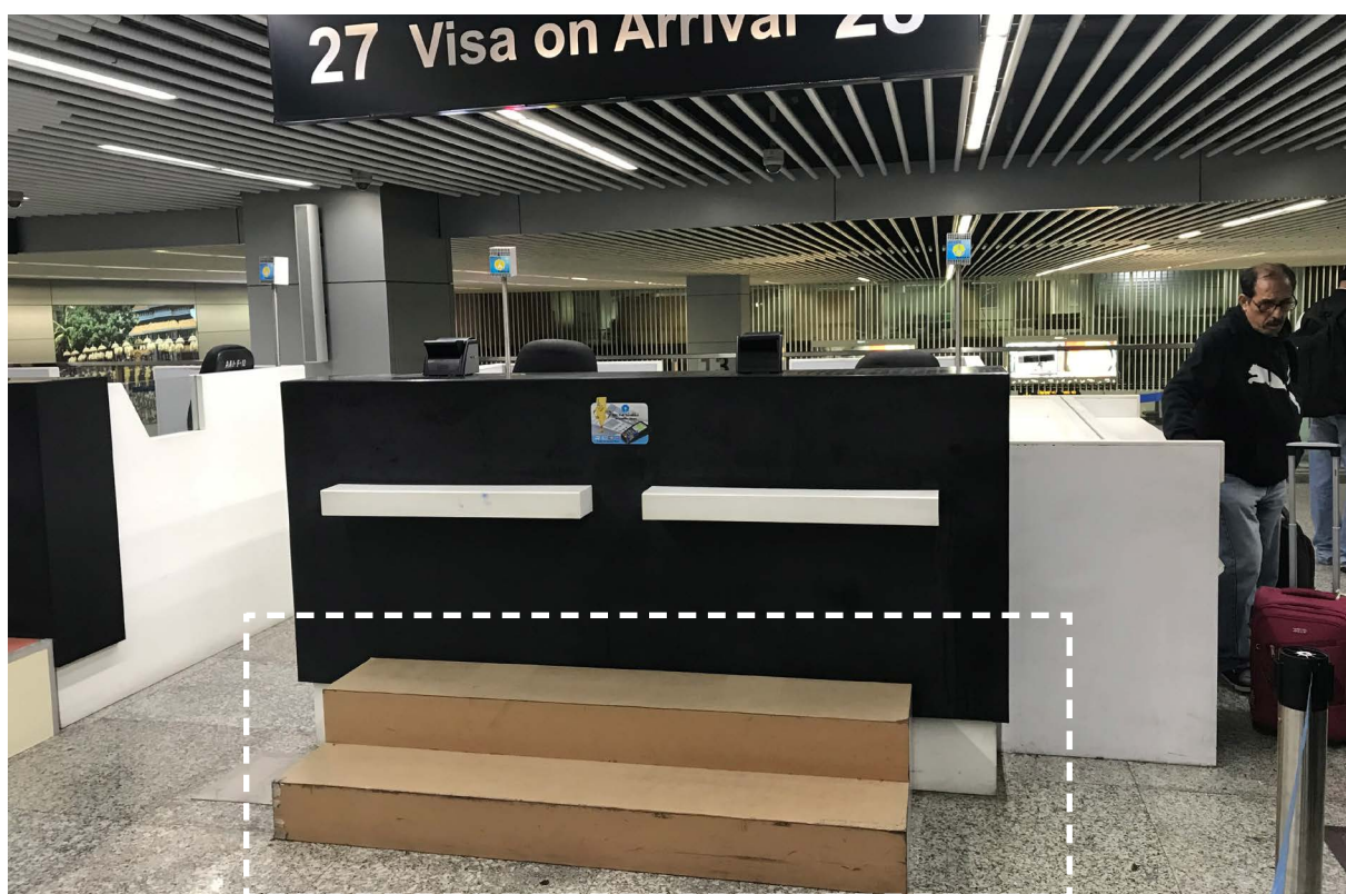
Image 2.25 Inaccessible counter heights
