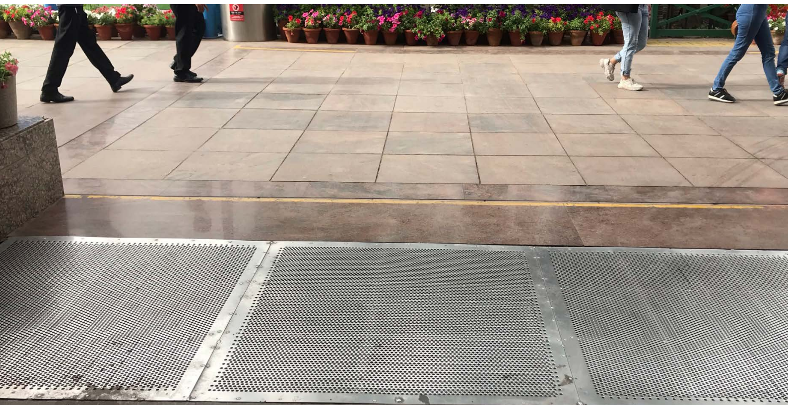
Image 3.12 Accessible grating details ( Perforated grating type) Photo Credits: Dr. Gaurav Raheja
