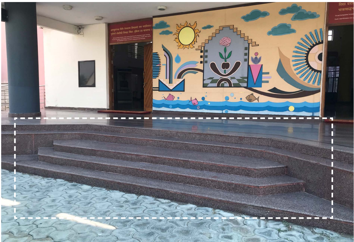
Image 2.3 Absence of adequate visual contrast in steps
