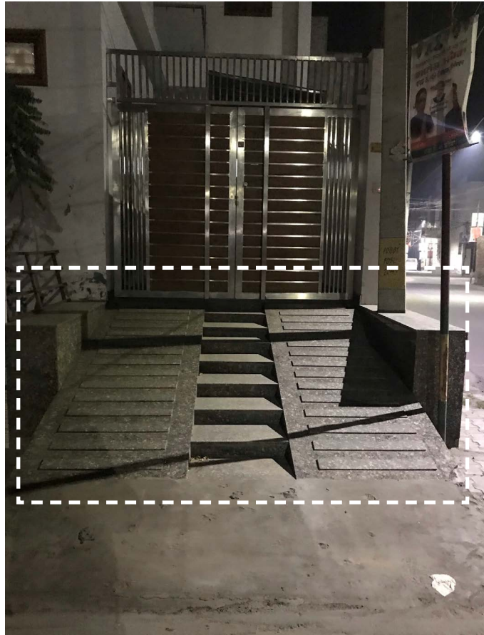
Image 2.14 Improper ramp detailing
