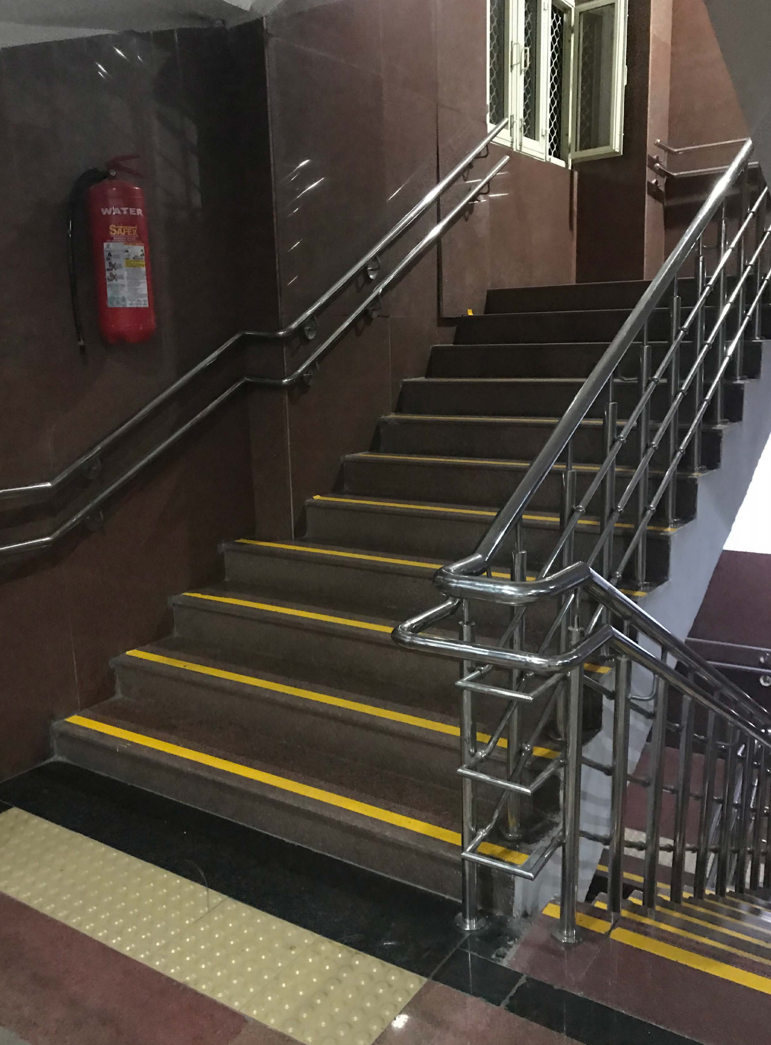
Image 5.13 Colour contrast on staircase Photo Credits: Dr. Gaurav Raheja
