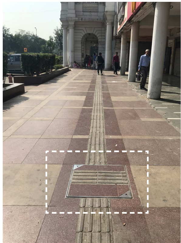
Image 2.20 Inconsistent laying of tactile guiding tiles
